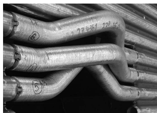
Fig. 2. The overlay welded opening of the membrane wall
