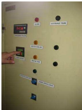
Fig. 3. Acid dilution supervision and control cabinet
