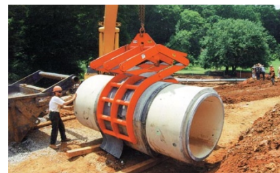
Fig. 1. Lifting of concrete pipes [3]
