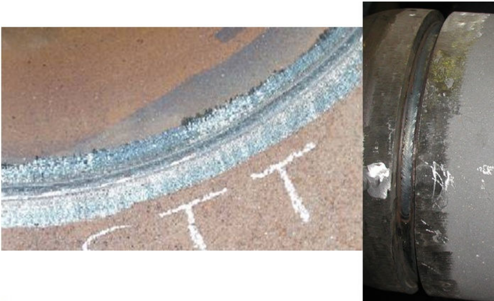
Figure 8. MAG-STT welding process in application at root pass on pipe chamber joint
