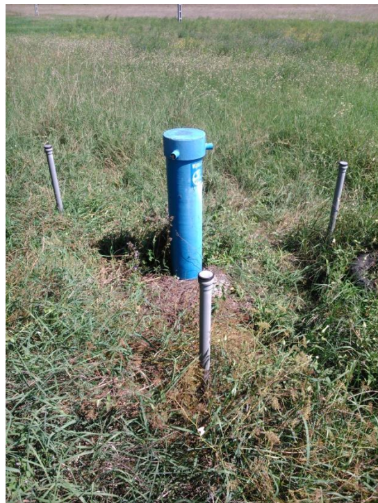
Figure 3. Three test holes next to a groundwater well
