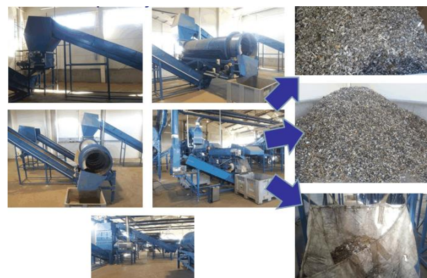
Figure 6. Separation-technology prototype at ALCUFER shredding-plant Fehérvárcsurgó, Hungary
