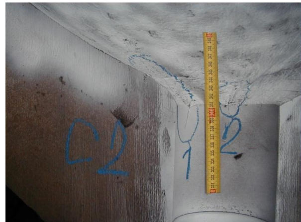
Figure 1. The crack in the throat zone at the bottom head - vessel segment C2
